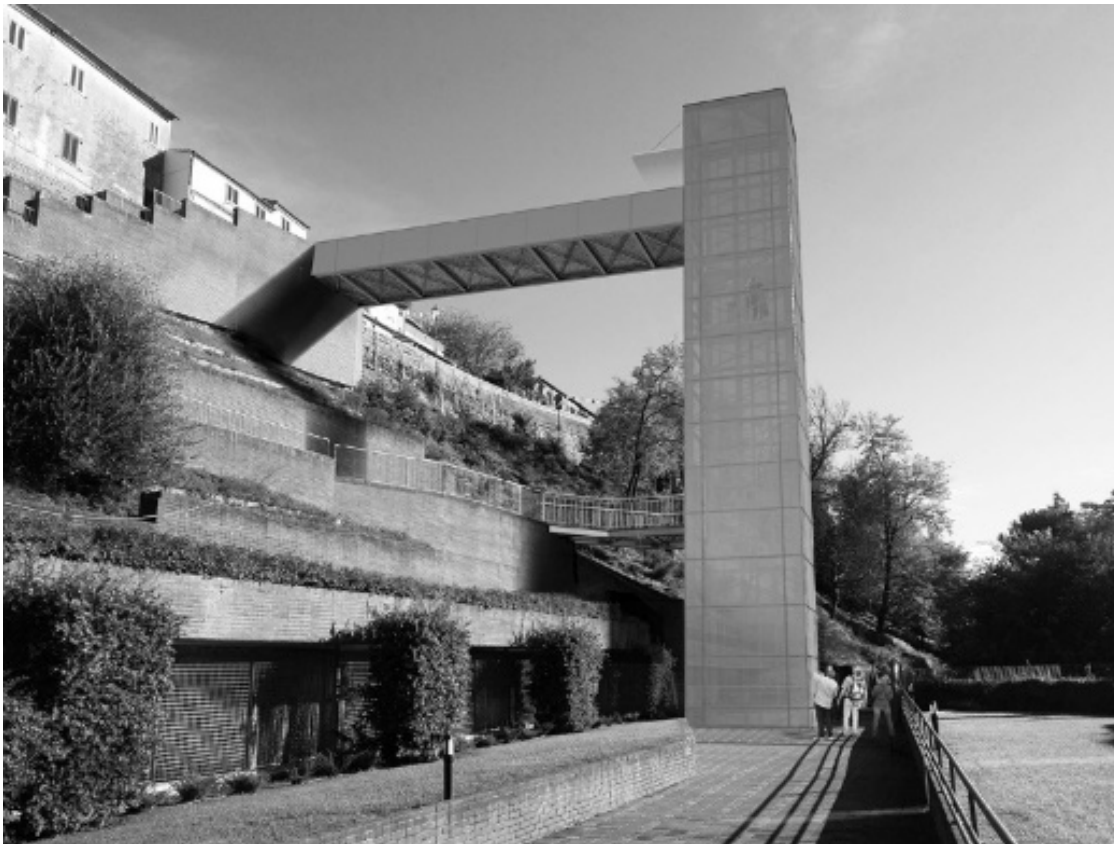
Figure 1. Rendering of the second lift in the municipal multilevel car park (designed by Alfonso Guiggi).
